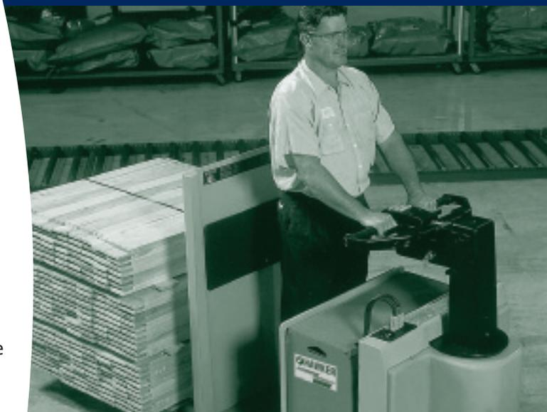
**No Watering**—Since the ENVIROLINK™ battery is a sealed battery, no water will ever need to be added, not for the lifetime of the battery. No watering. No room for over/underwatering error.
